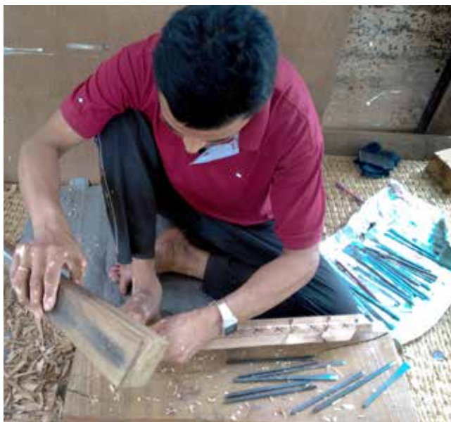
Char Narayan Temple | May 10, 2016 Woodcarver Hari Prasad replicating one of the missing pieces from the main doorframe.
