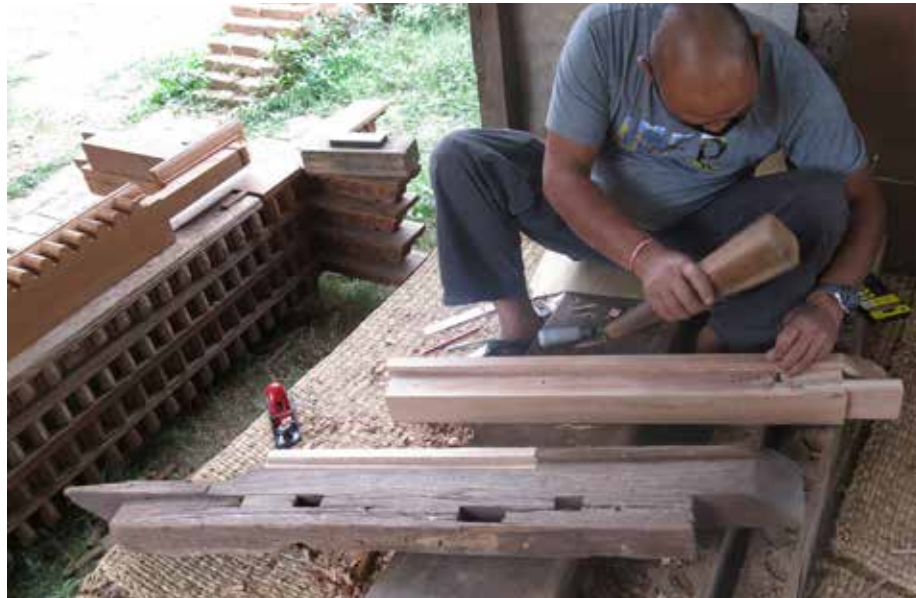
Char Narayan Temple | May 05, 2016 Woodcarver replicating the missing purato (outer frame) of the door.
